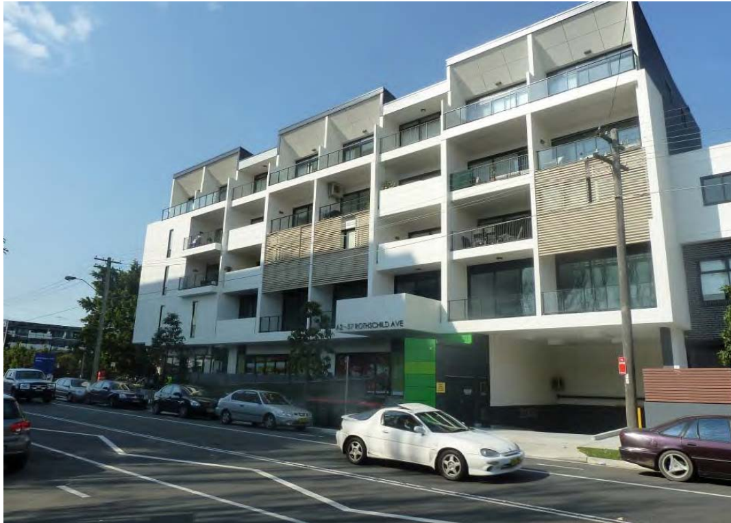
Figure 4: Existing residential building opposite the site – Rothschild Avenue
